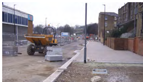
■ Construction works in progress
