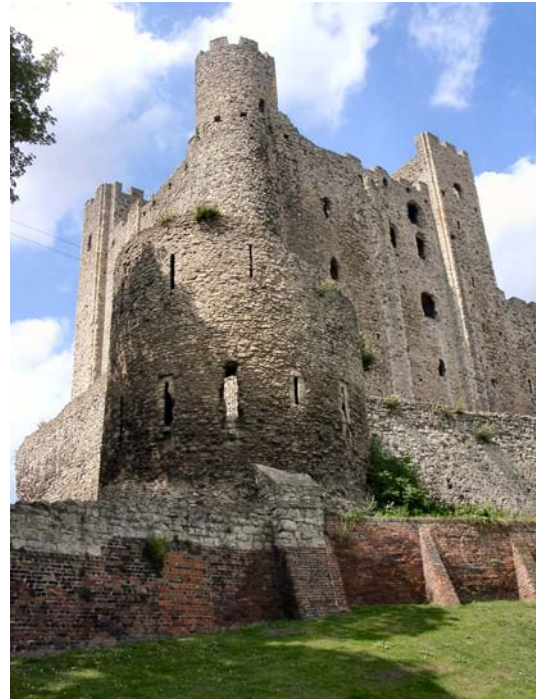
The (rebuilt) corner of the keep and bailey wall attacked by King John
