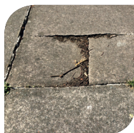
Broken slabs
