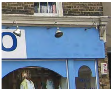
These large swan-neck lights have been knocked and broken. They look clumsy, not classy.
