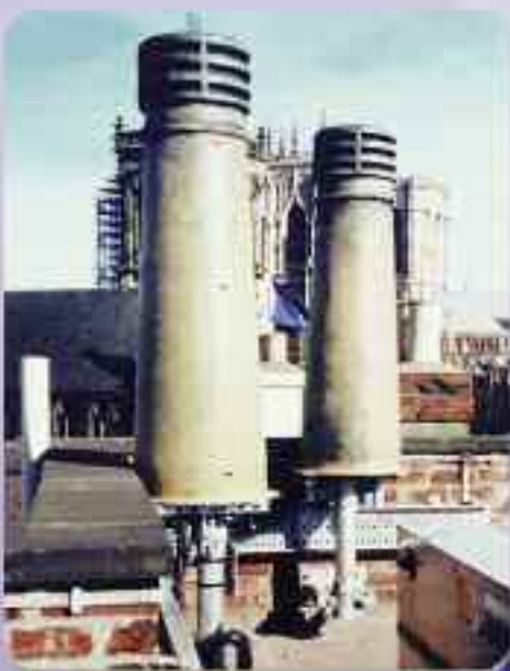
Antenna concealed in GRP chimney pots close to York Minister
