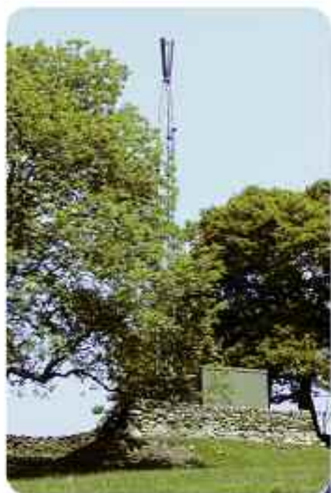
Lattice mast in the Lake District that uses trees as screening
