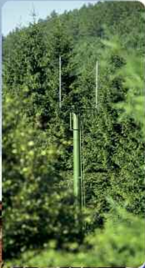
Monopole mast painted green with antennas
