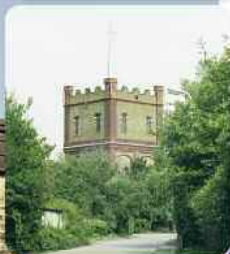
Antennas painted to reduce contrast
