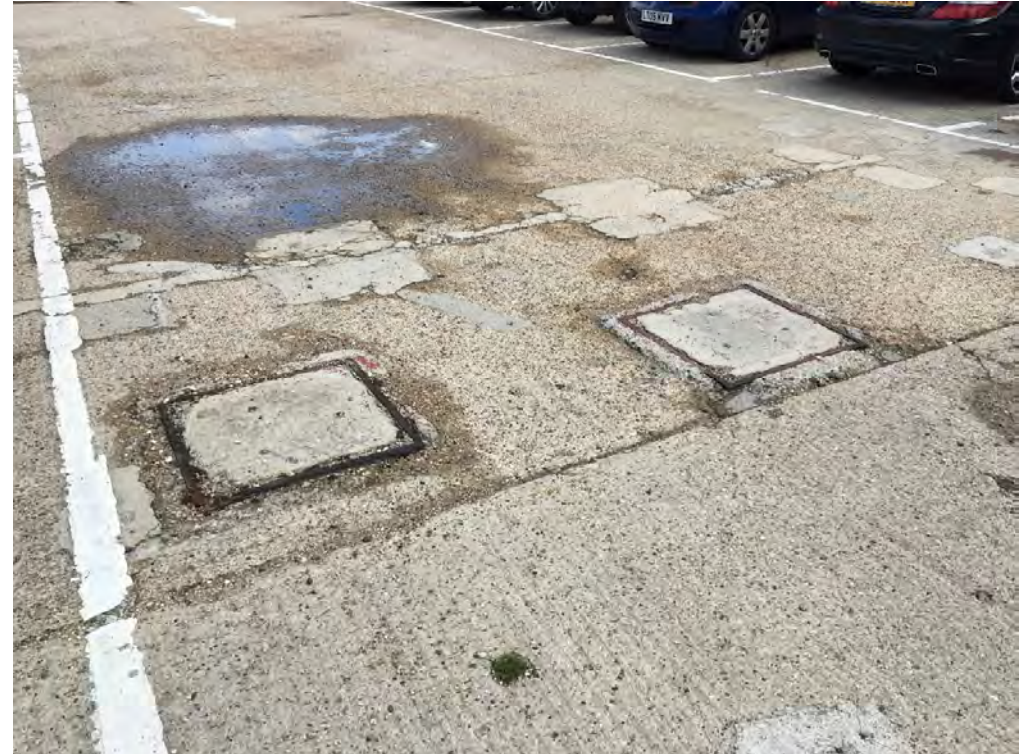
Photo 10: Concrete area in east of Area 2
