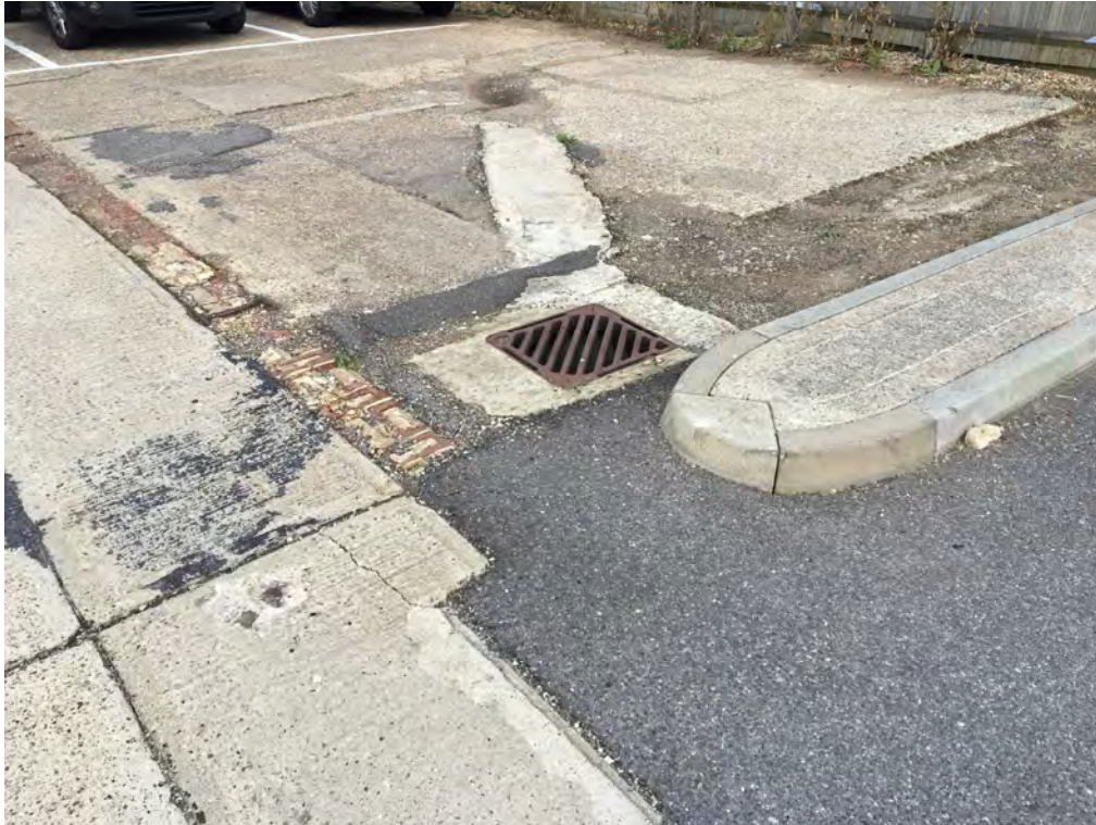
Photo 11: Concrete and drainage in north east of Area 2
