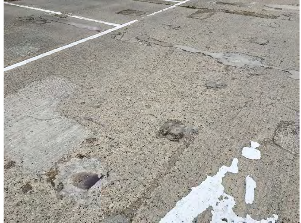
Photo 8: Concrete area in east of Area 2
