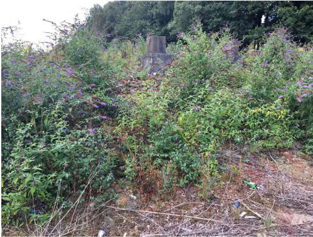
Photo 5: Concrete structures at north of raised platform area
