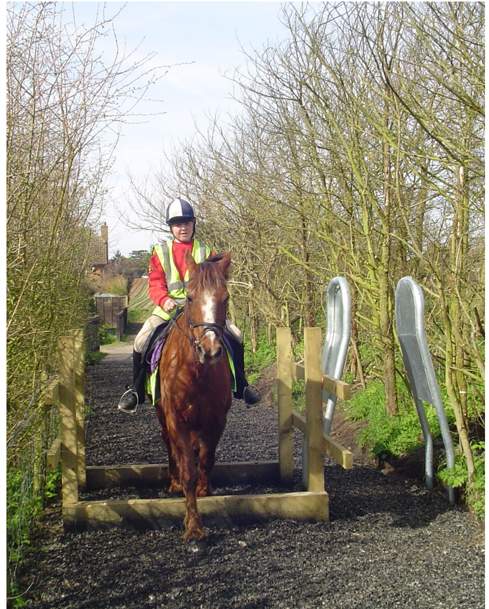
Improvements to public rights of way for equestrians – new rubber crumb path near Cliffe.
