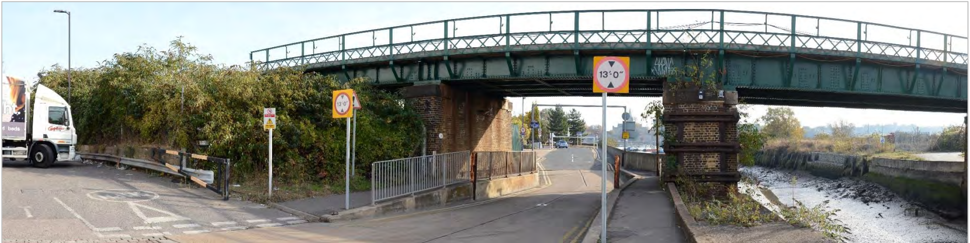
Figure 2-8: Phase 1 site from the railway embankment bridge to the west, looking along the western boundary of the site, adjacent to Jane's Creek
