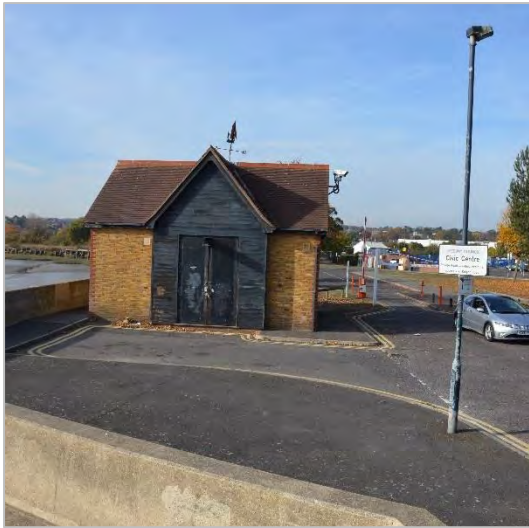
Figure 2-11: Pump House on the Phase 1 site
