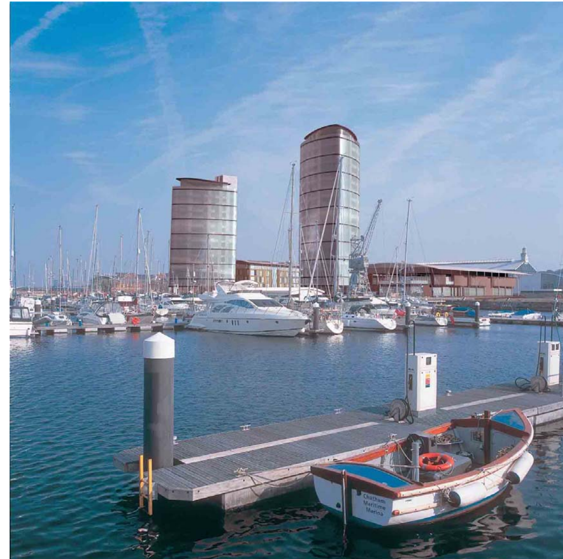
15 and 19 storey towers on the dock fingers at Chatham Maritime- Dockside Outlet Centre prominent in the background.
