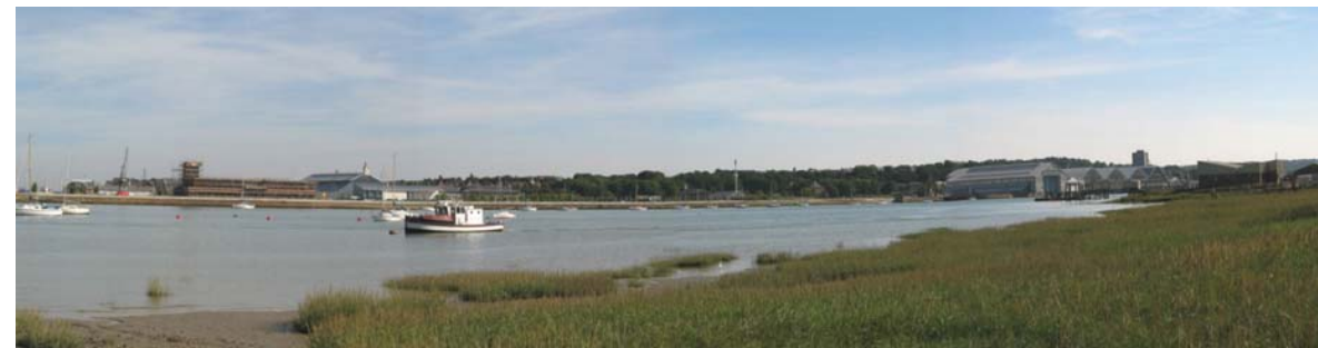
View from Upnor. The covered slips of the dockyard are prominent on the right. The interface land is the currently undeveloped area in the centre of the picture. The back drop of Amherst Hill is a key feature.
