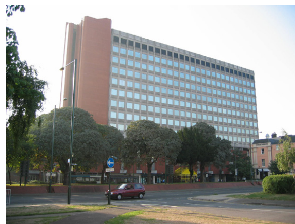
Mountbatten House, one of Medway's tallest buildings that overlooks the waterfront area
