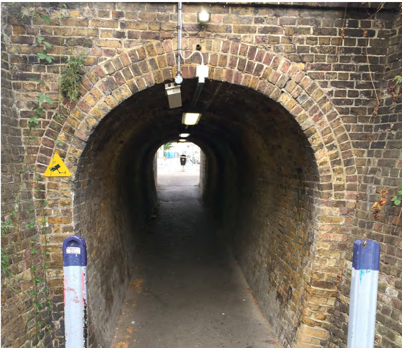
Pedestrian underpass to Strood Station from Station Road
