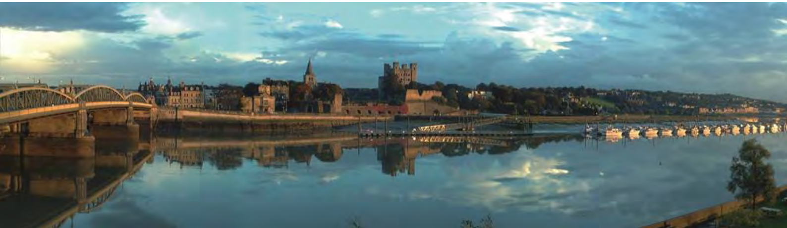
View from former Civic Centre site across to Rochester
