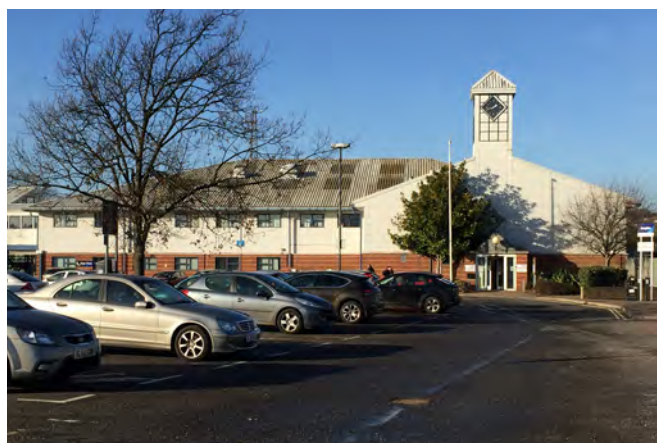
Former Civic Centre Site
