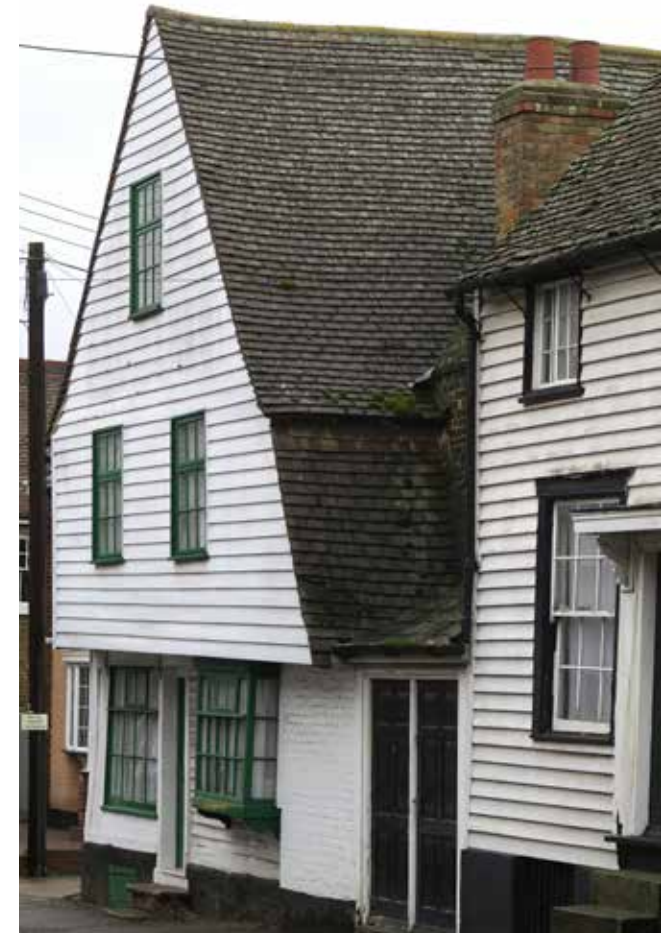
Figure 12: Listed gabled houses with jettying upper floors on Church Street
