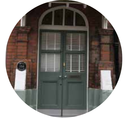
PAINTED DOOR FRAME
