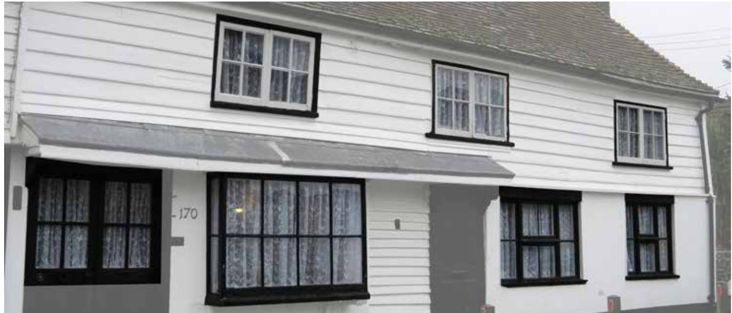
Figure 45: Listed building with historic window features.
