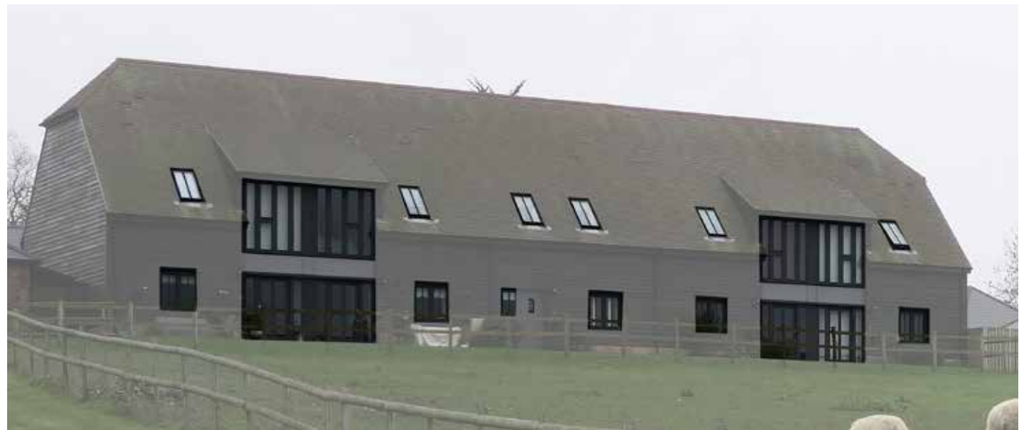
Figure 46: Contemporary building using variations in building rhythm and proportions to articulate the horizontal mass of the building
