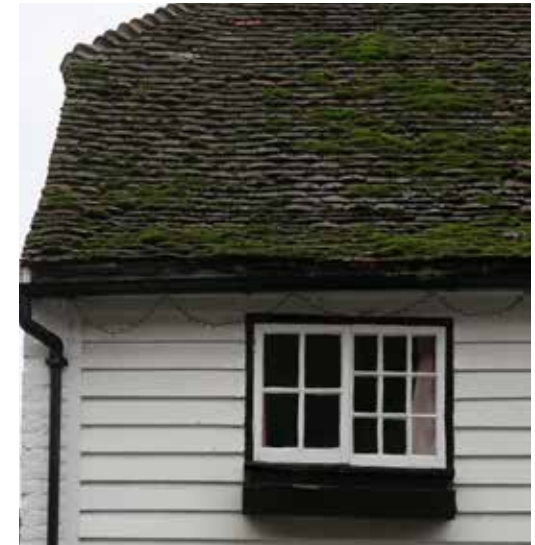
Listed building with a half-hipped roof with clay plain tiles and white weatherboarding.
