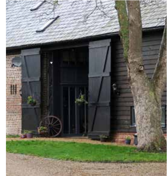
Renovated agricultural building with brick and black weatherboarding
