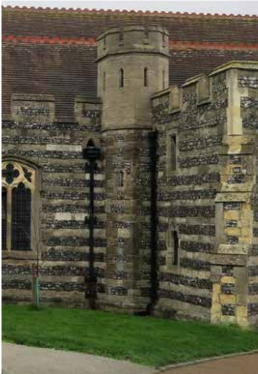
Churchyard and Church of St Helen with a crenelated parapet and walls composed of an alternation of flint and stone.
