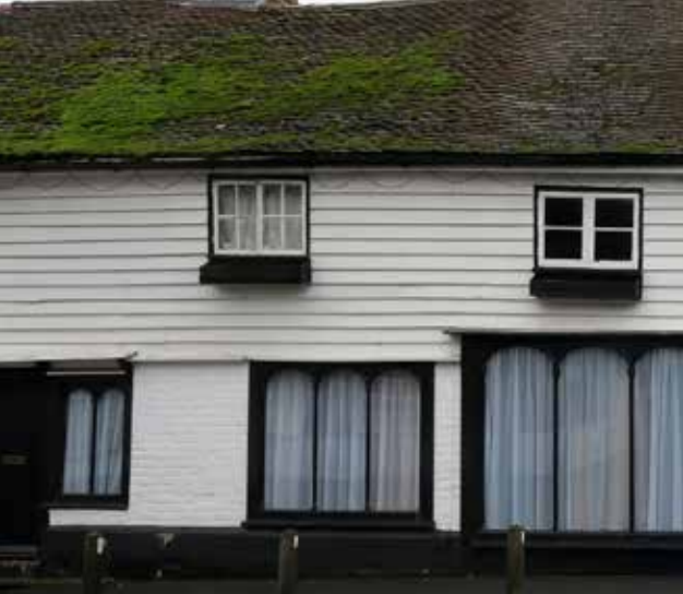
Listed buildings with clay plaintiles roofs, white weatherboarding, and black window and door frames.
