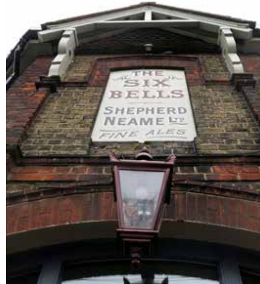
Six Bells corner building with red and grey brick façade.
