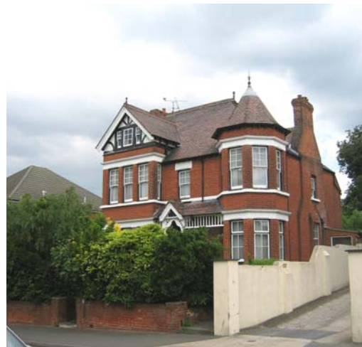
Decorative Brickwork, 43 Maidstone Road
