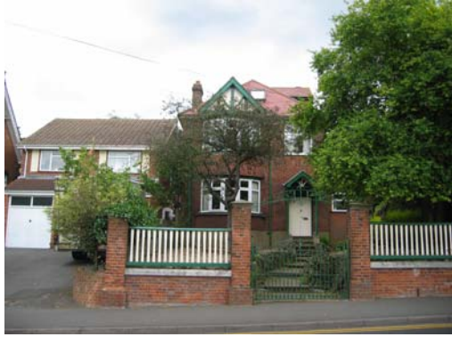
1930s Housing, showing unusual timber fencing
