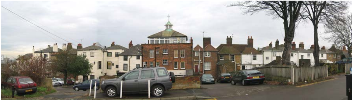
Rear of 2-28 New Road
