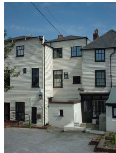
Rear of 8-10 New Road
