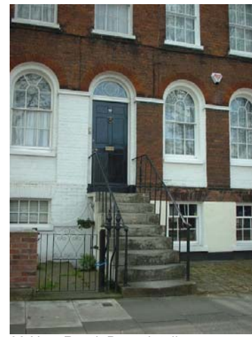
38 New Road, Door detail
