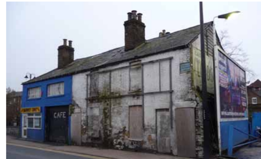
25-31 Corporation Street, buildings of little architectural merit
