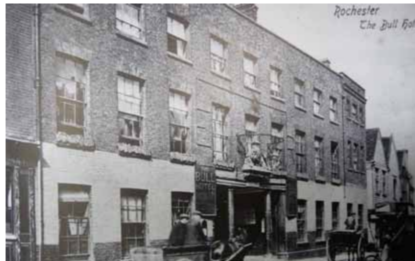
The Bull C.1910, alterations including removal of detail and painted brick
