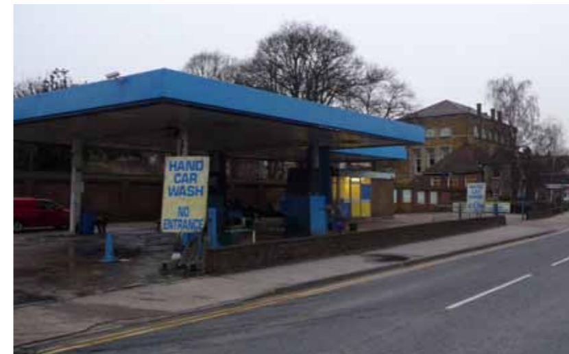
Vacant, former Petrol Station, Corporation Street
