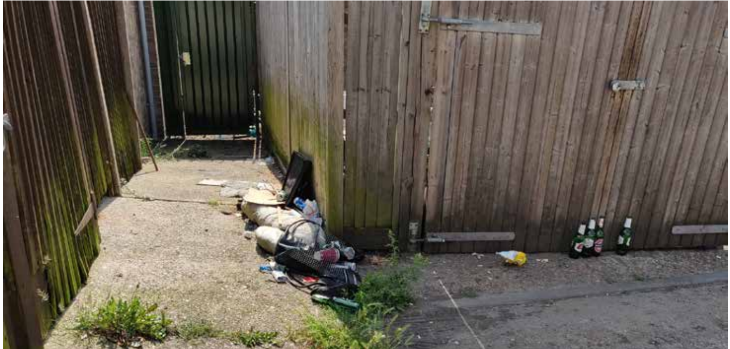
Figure 31: Photo of a recessed gate showing an accumulation of detritus.
