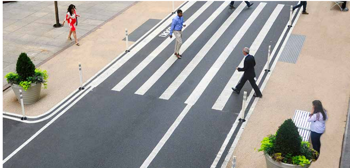
Figure 26: Painted kerb buildouts with movable planters at a mid-block crossing in New York, United States. Note: complementary delineation devices such as wider tactile paving areas are likely to be required to guide visually impaired pedestrians (© New York City Department of Transportation).
