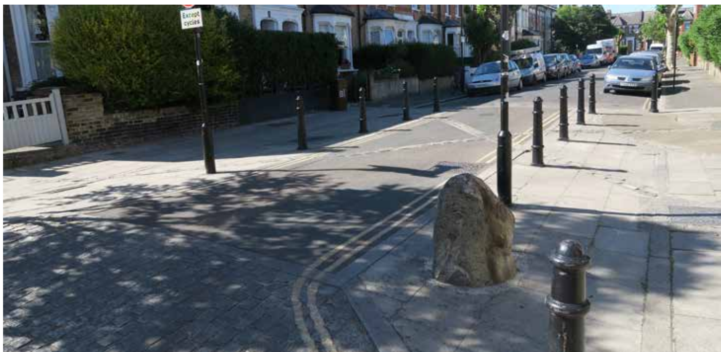
Figure 22: Raised entrance to a residential street in London combined with kerb buildouts at corners.
