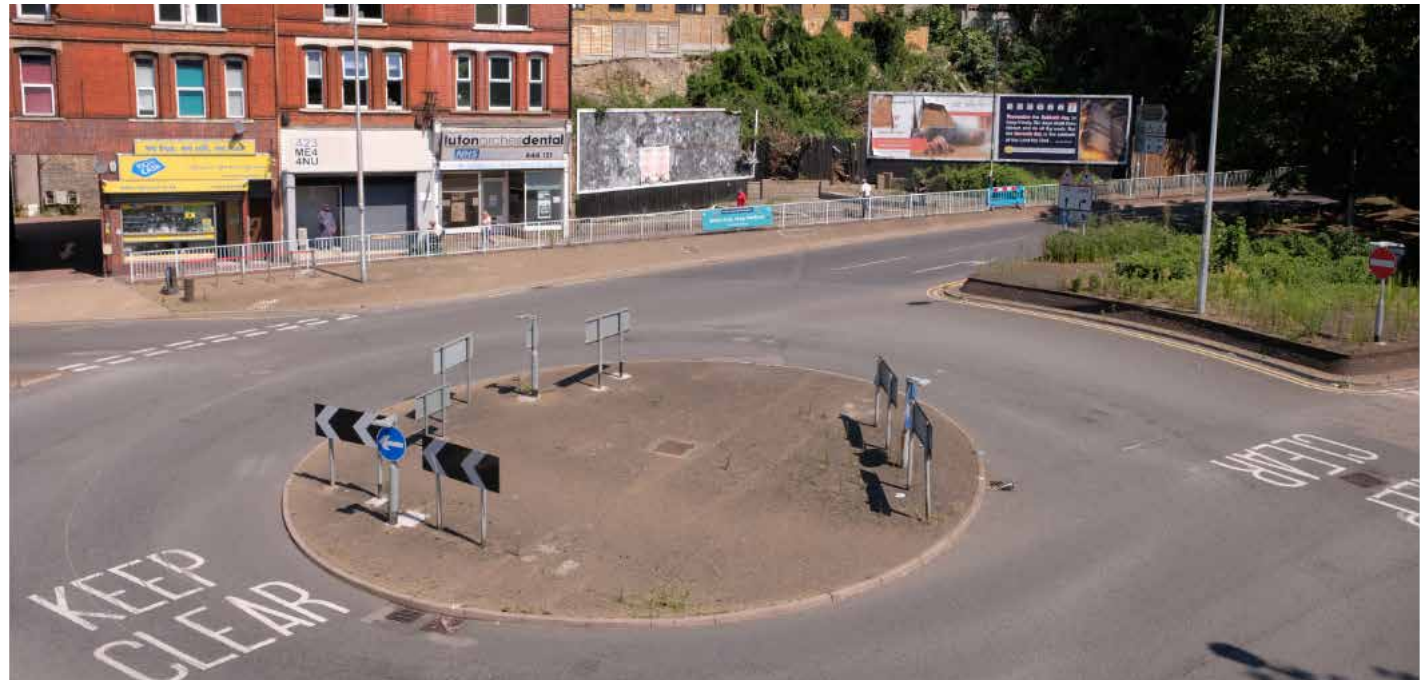
Figure 24: The A2 junction and roundabout must be reconfigured to improve safe at-grade pedestrian access and reconnect Luton Road to the centre of Chatham.
