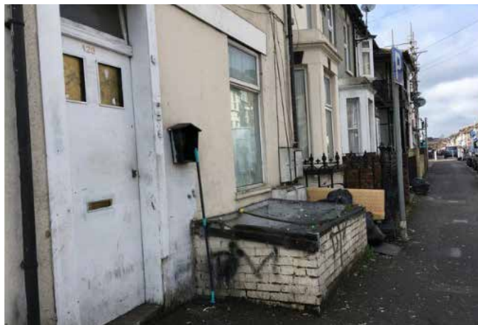
Figure 15: Poor investment in properties, Luton Road.
