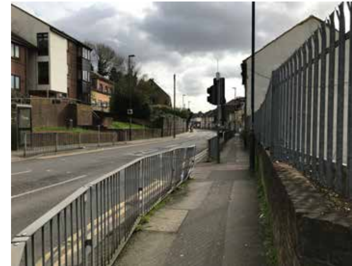
Figure 6: Poor pedestrian environment along Luton Road.
