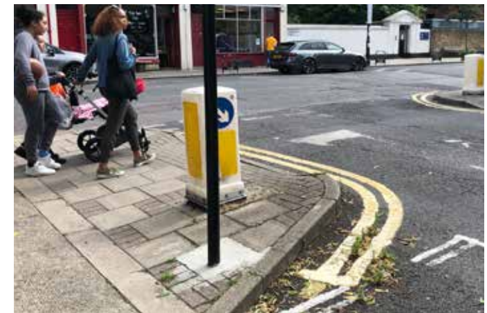
Figure 23: Left: a kerb buildout used to shorten pedestrian crossing distances and calm traffic. Right: a buildout with street greening and a double kerb to prevent vehicle overrun. Note: tactile paving areas are likely to be required to guide visually impaired pedestrians.
