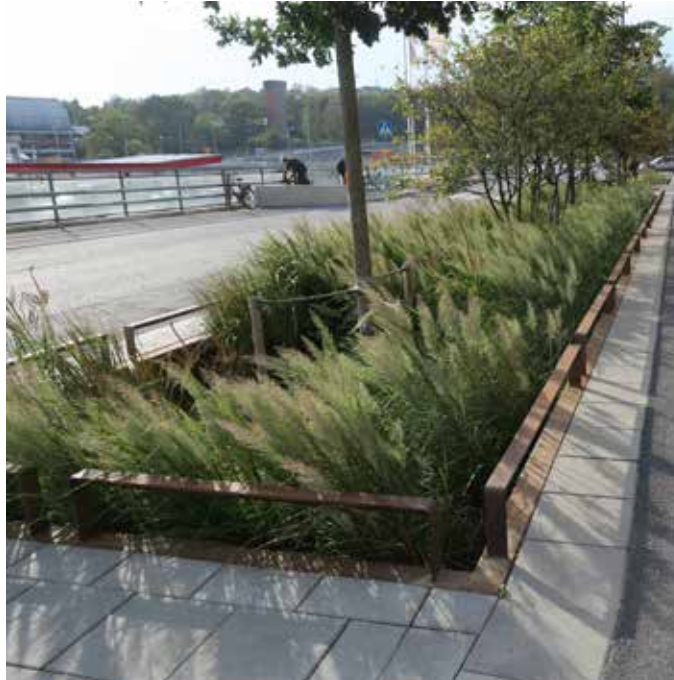
Figure 36: Roadside swales with low-level planting and new trees in Stockholm, Sweden (left) and London (right).
