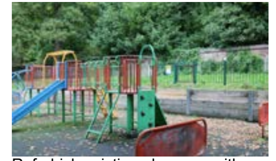
Refurbish existing play area with additional play equipment
