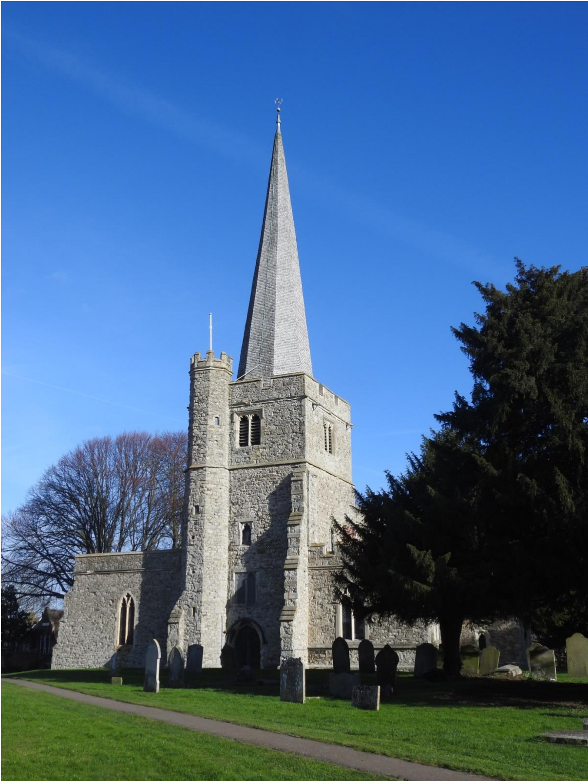
Hoo St Werburgh Parish Church (Grade I Listed), part of the area's rich and varied built heritage.
