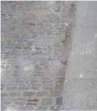
Porphyry/granite setts and cobbles with granite kerbstones
