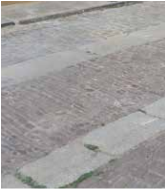
Porphyry/granite setts and cobbles with granite kerbstones
