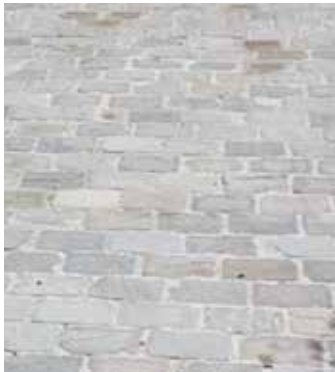
Natural stone Granite or porphyry setts
